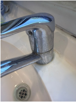
Image of leaking basin tap.
